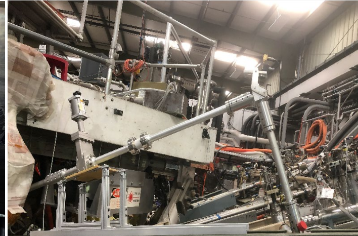
Top Launch waveguide run with switch to select radial or top launch
