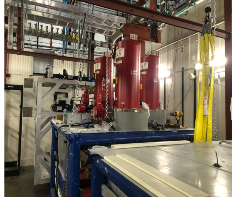
Klystron installation underway outside DIII-D radiation shield wall
