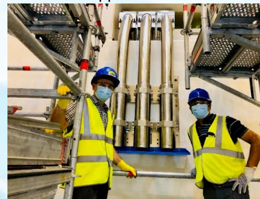
NFM#7 Support Frame Installation
