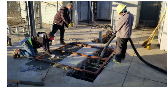
Boost Transformer foundation
